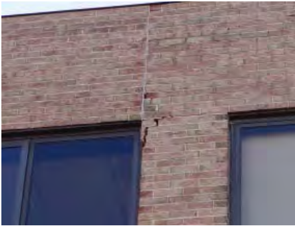
Figure 6.19: Spalling exterior brick walls
