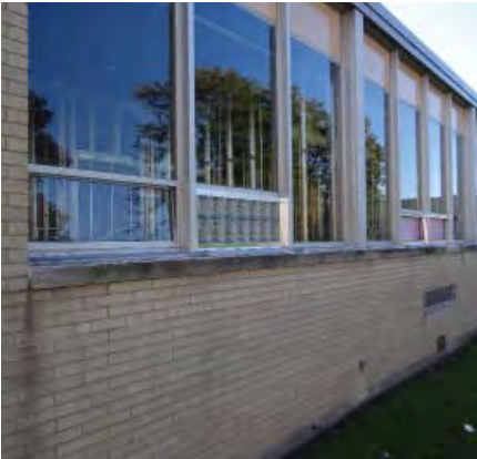
Figure 6.20: Inefficient single-pane glazing
