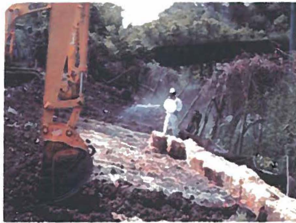
During remediation: Excavation along fence line, using water for dust control
