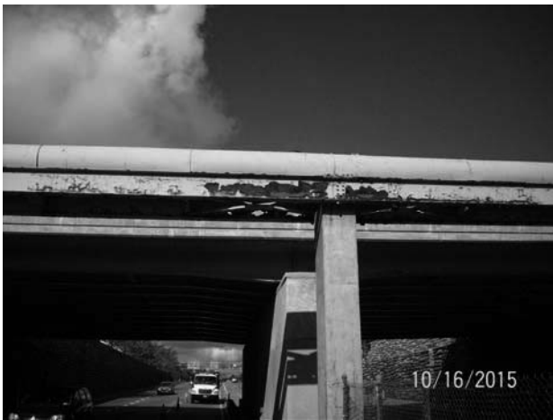
East side of bridge at Pier
