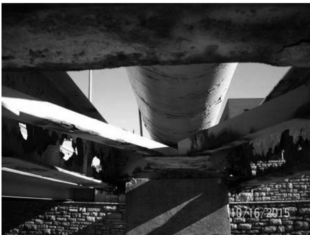
Looking north between girders near pier
