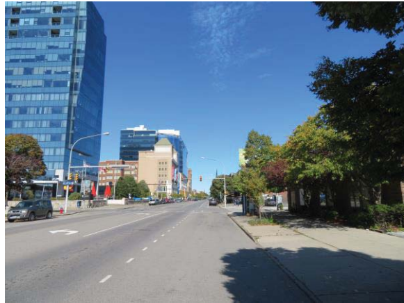
Delaware Avenue Viewing North
