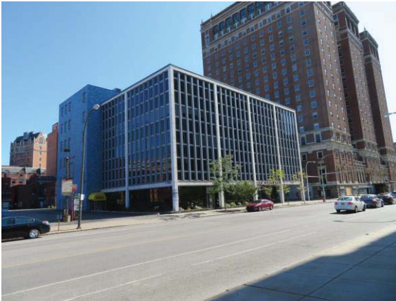
135 Delaware North & West Elevations
