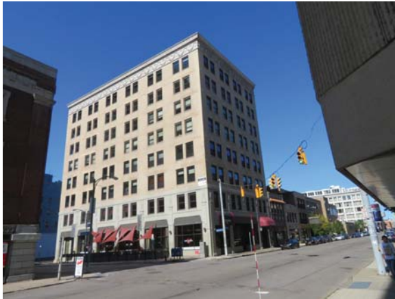
South and East Elevations
