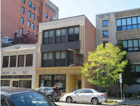
Front View – Franklin Street
