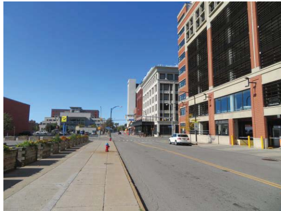
West Huron Viewing West
