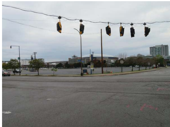
142 Perry Viewing Southwest
