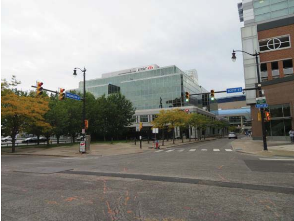
Washington Street Viewing South
